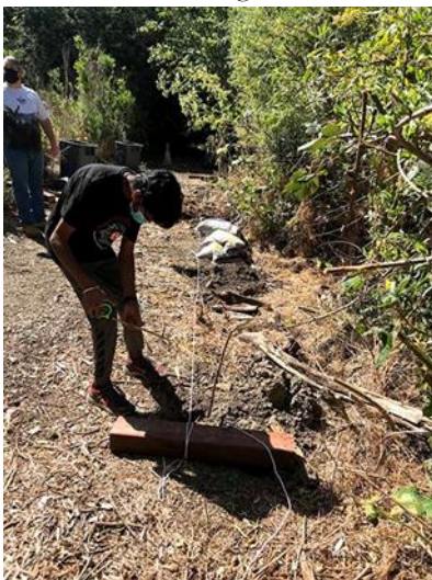
Trail with Retaining Wall – Tule Ponds
