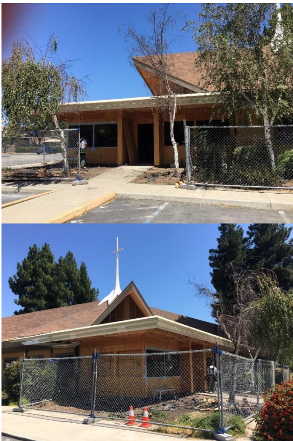
FIRE REPAIR PROGRESS 7-30-2020
